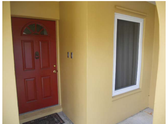
IMPACT RATED WINDOW AND UNPROTECTED FRONT DOOR
