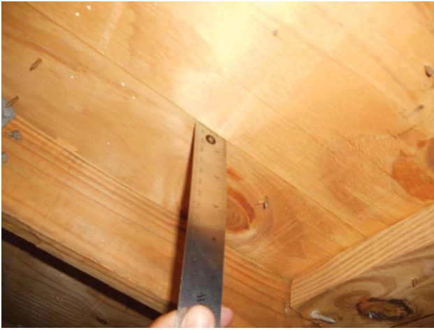
ROOF DECK MEASUREMENT
