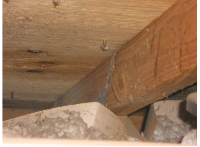
Roof to Wall Attachment: SINGLE WRAPS
