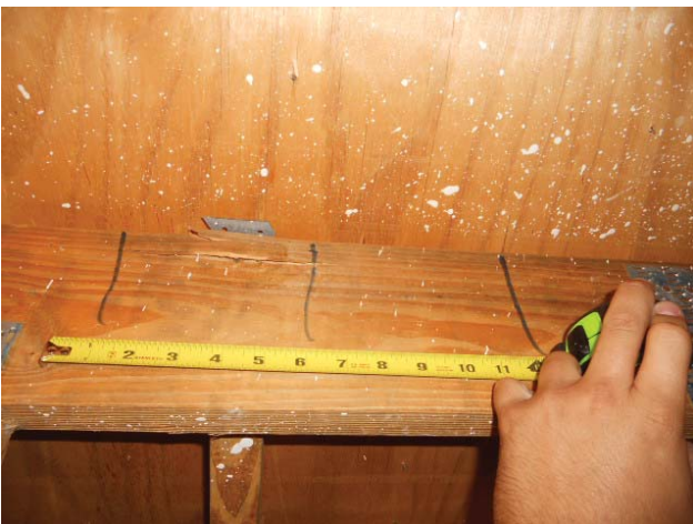
Roof Deck Attachment:- 6" NAIL SPACING
