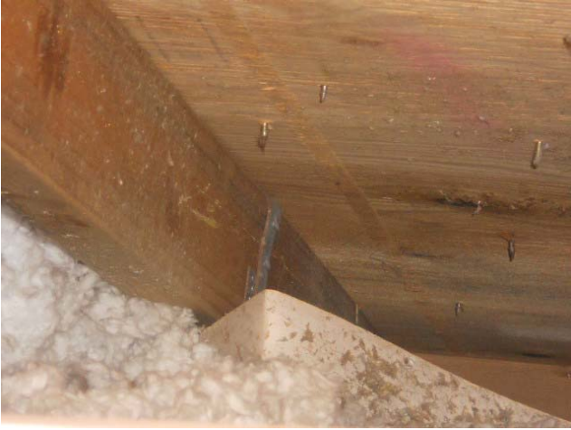
Roof to Wall Attachment: SINGLE WRAPS
